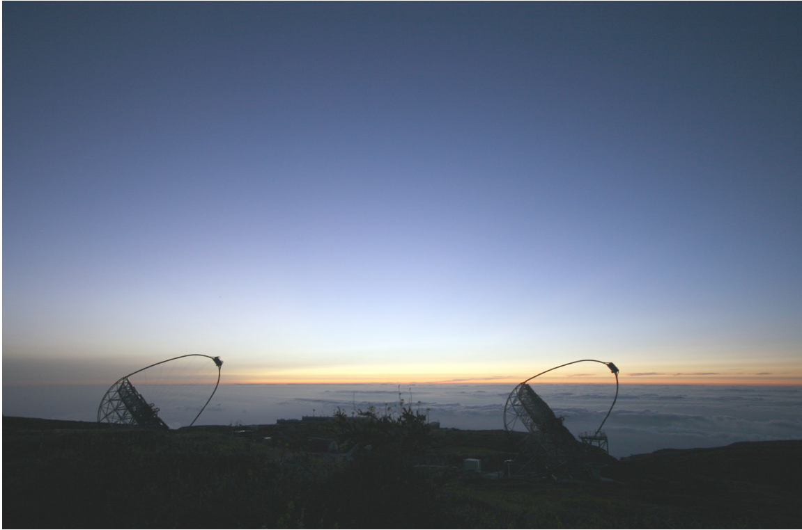
Figure 3.6 The MAGIC telescopes at the Roque de los Muchachos Observatory in La Palma island, as seen in the sunset from the East. Each MAGIC telescope is a single dish mirror of 17 m diameter, the largest collecting mirror in the world to date. They are 85 m far from each other following sensitivity Montecarlo studies.
