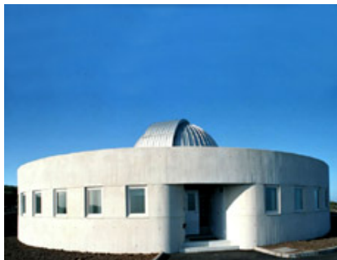
Figure 27: Building of the IAC-80 telescope. Credits: IAC webpage.
