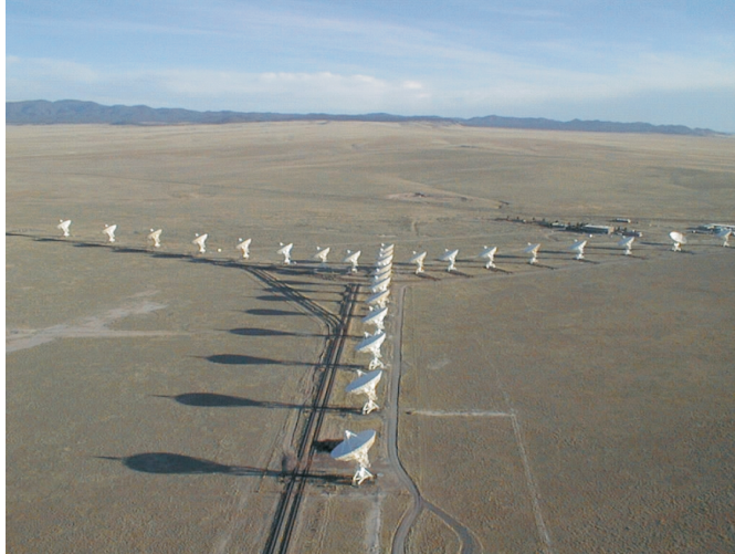
Figure 2.4: An aerial view of the Very Large Array showing the iconic VLA’s Y-shape that give its highest resolution capability. Credit: NRAO/AUI/NSF
